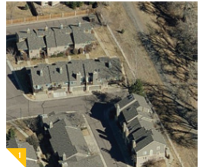
FIGURE 1 A Microsoft Virtual Earth aerial image of a development Vibrant Solar is evaluating for optimum solar access. X marks the southern facing rooftops.
