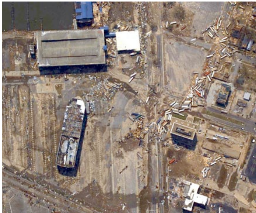
Hurricane Katrina image captured with Trimble DSS RapidOrtho; courtesy of NOAA/NGS.
