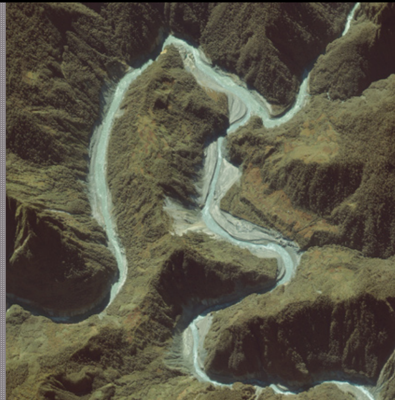
Figure 2 This image was captured in November 2000, after the flooding from a landslide that occurred in June 2000. Three bridges are missing in this image. The team used an improvised cable-crossing at the location of "Bridge #3," which was probably not yet constructed when this image was taken.
