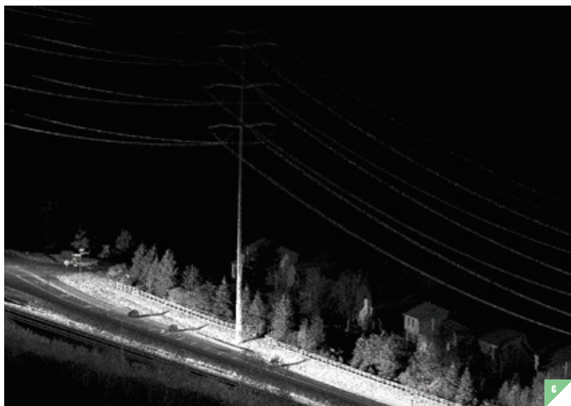
▲ FIGURE 6. Point cloud of power lines. Courtesy of Woolpert.
