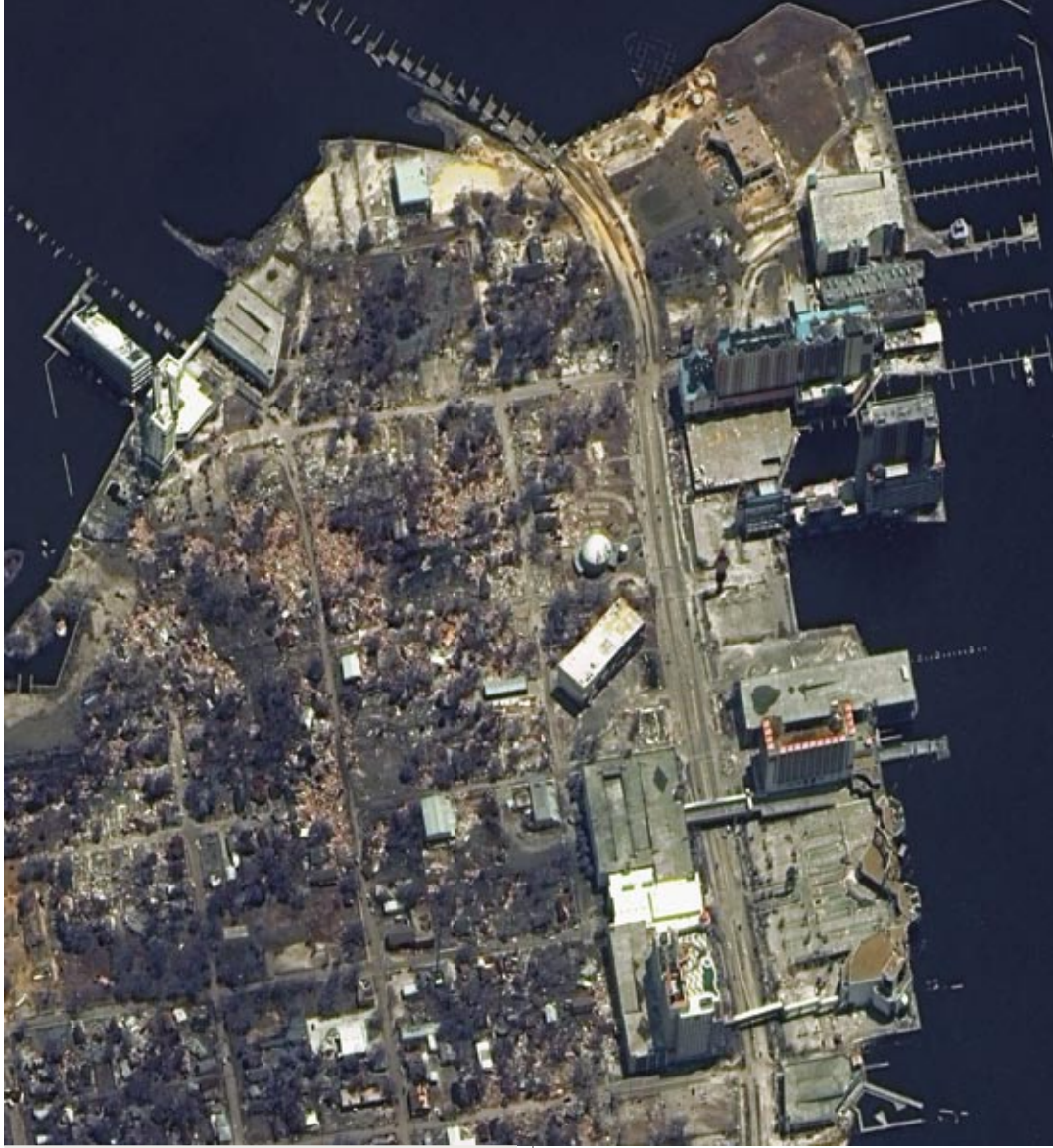
Waterfront in Biloxi, Miss. following Hurricane Katrina, one of the most devastating storms in the U.S. in decades (Courtesy of Digital Globe).
