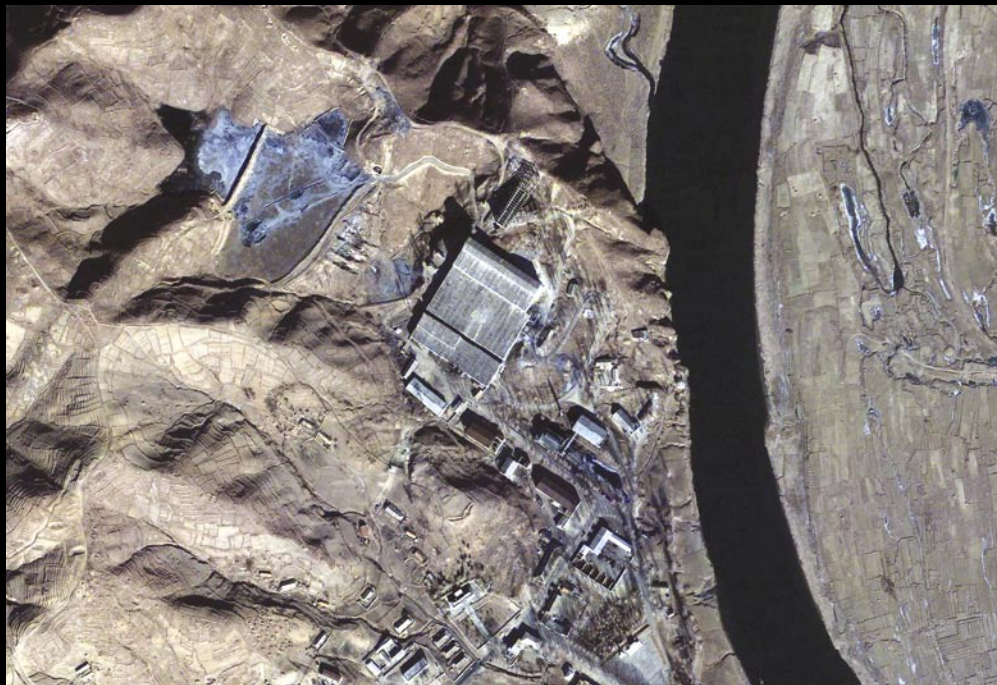
FIGURE 2 QuickBird photograph of Pakch'on Uranium Concentration Plant, acquired December 13, 2003.
